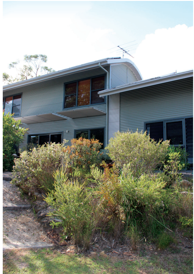
Above: Residential property with a well designed and maintained bird friendly garden that meets APZ requirements
